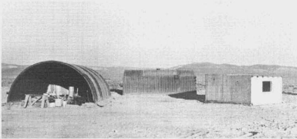
Fig. 6.2 Test Structures in Cleared Area (L to R: Bldgs 1, 2, and 3)
